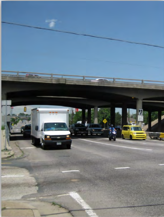
Kipling Street under I-70 bridges
