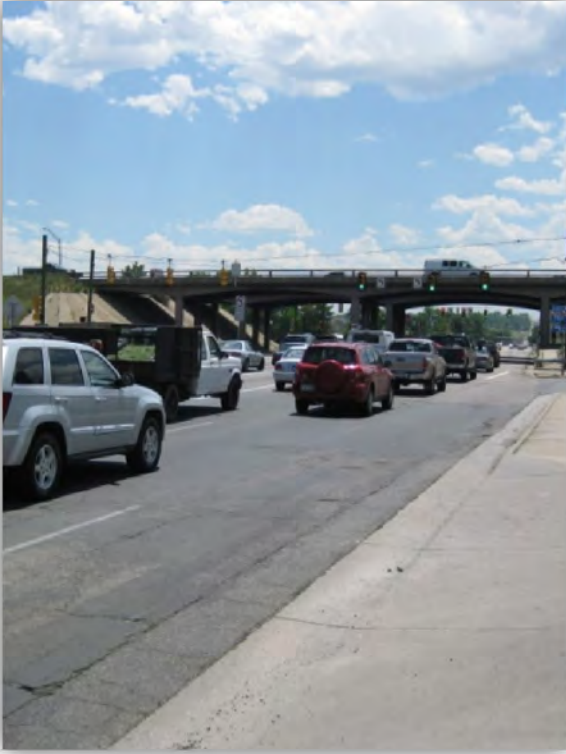
Kipling Street at eastbound I-70 ramps intersection
